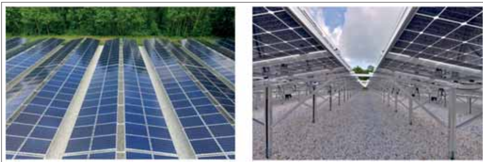
Figure 10. Bifacial 400kWp system from Tempres with East/West orientation [26x]. The white gravel results in an albedo of 40%. Left picture: View from above; Right picture: View onto the back of the bifacial modules.
