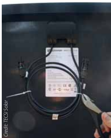
Figure 12. Removing standard factory installed wire ties
